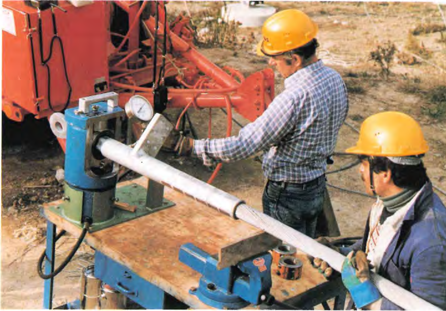
Fig. 20 Pressing of the compression dead-end clamp, pressing force 1500 kN
