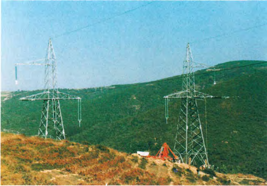
Fig. 22 Dead-end insulator sets at the terminal towers
