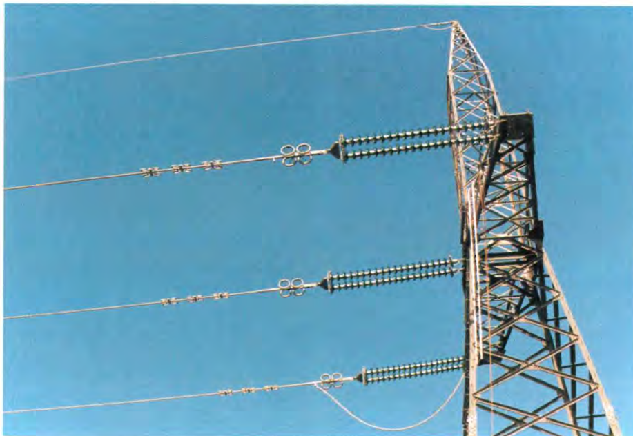
Fig. 25 Tension tower of the crossing with the phase conductors strung
