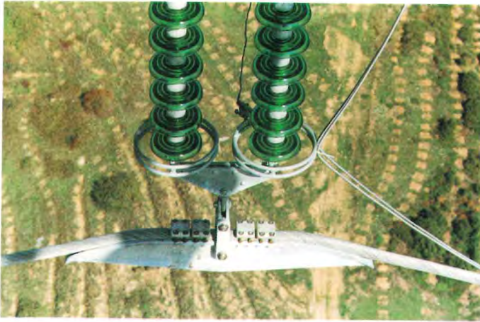
Fig. 14 Saddle-type suspension clamp installed
