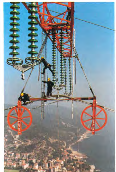
Fig. 3 Conductor blocks and suspension saddle
