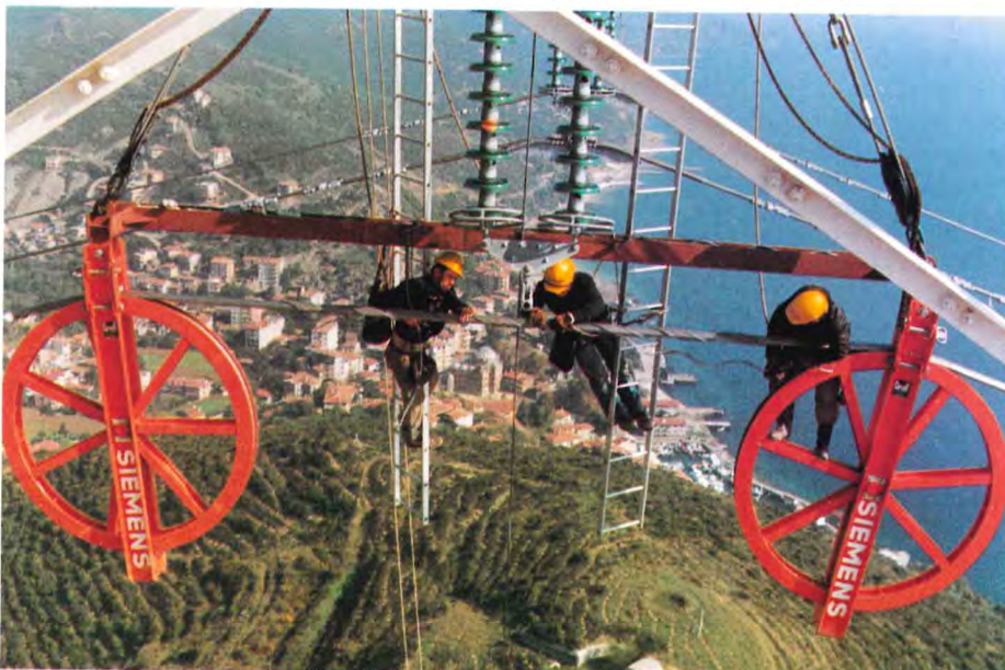
Fig. 15 Installation of armor rods
