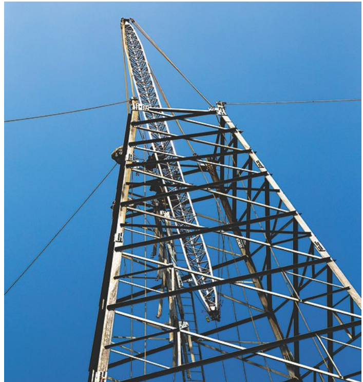
Lifting load is indicated in 3 positions: pos.1 vertical, pos. 2 with 20 degree inclination installed in the tower center, pos. 3 with 20 degree attached to a towerleg. Please note: operation of the Ginpole always requires some inclination.
