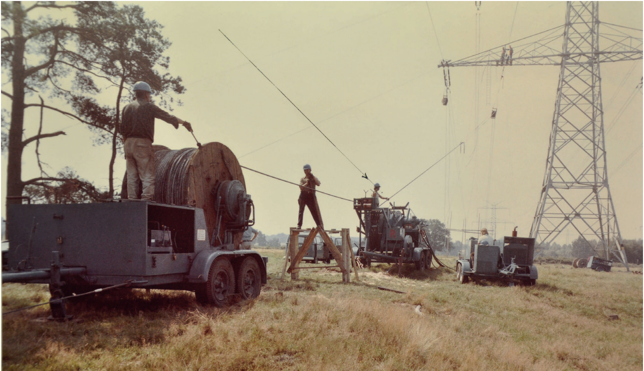
ZECK Puller-Tensioner WB 1500 in operation
