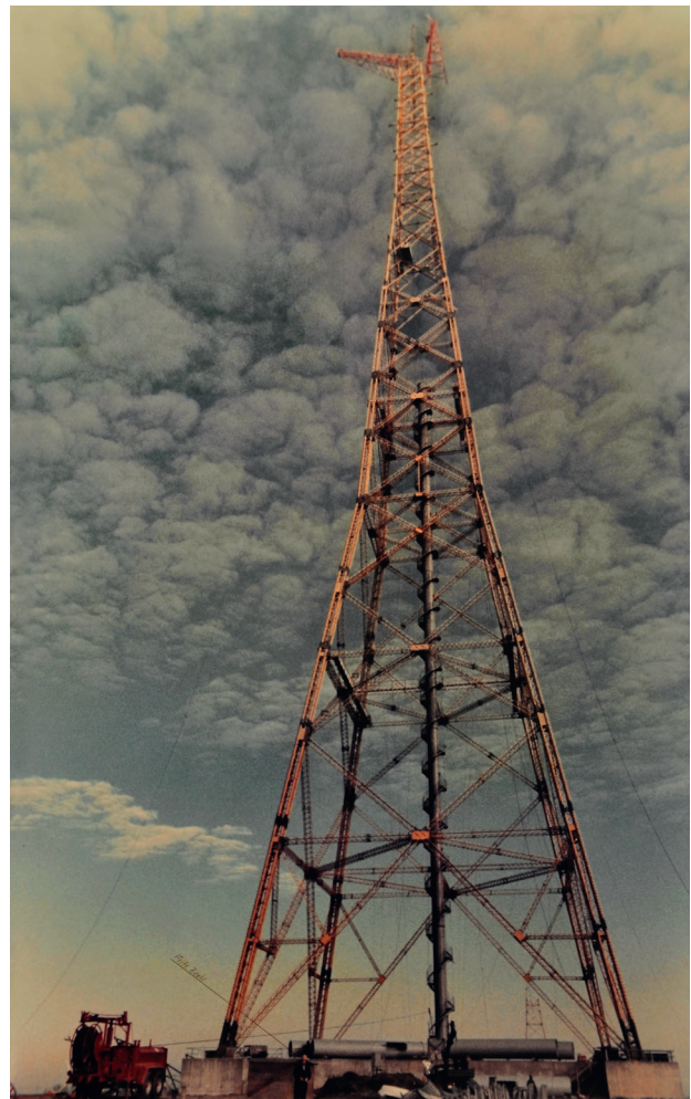
Overhead transmission line tower of the Elbe crossing with spiral staircase inside, 227 m high
